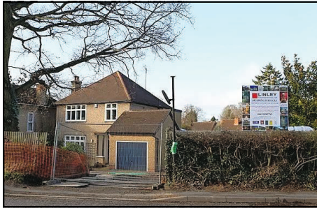
The property where a builder was killed by a falling wall
